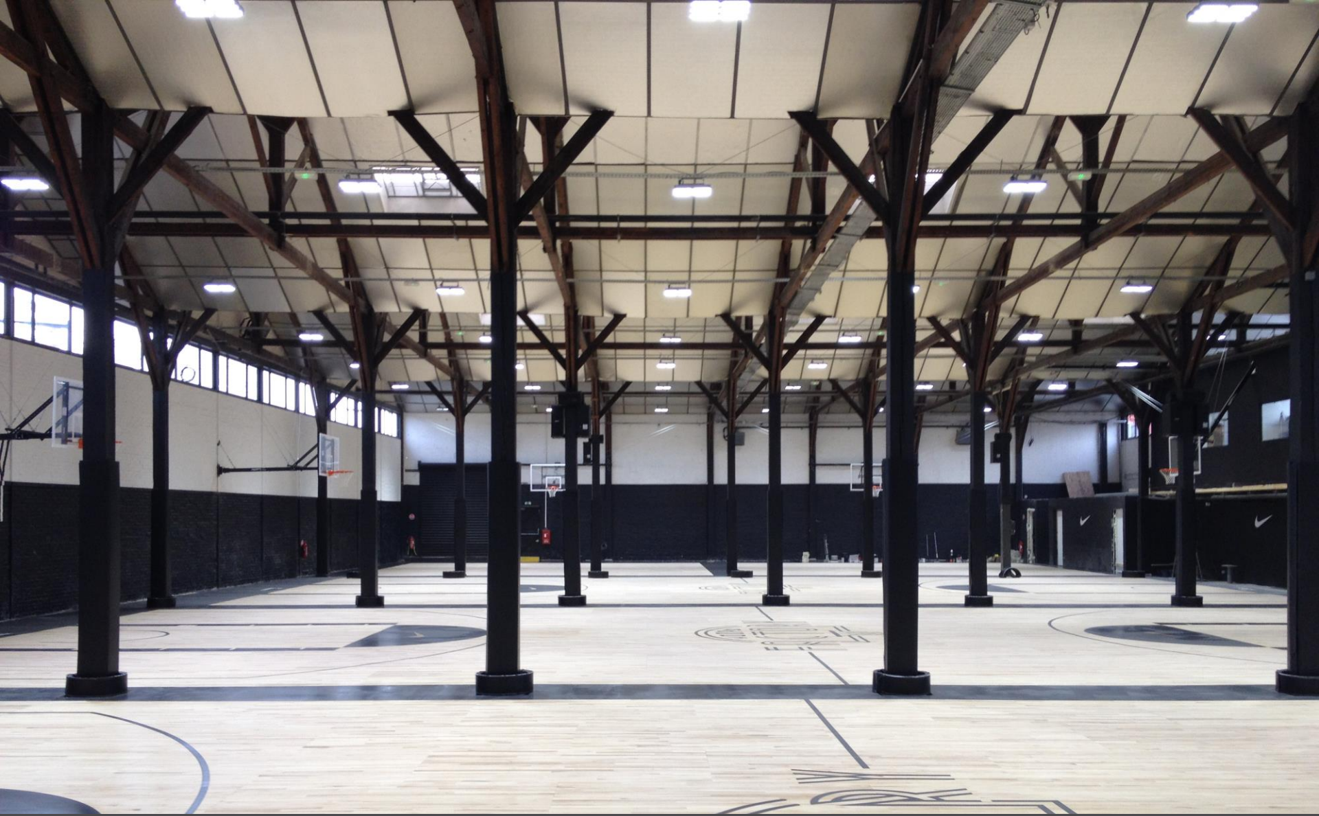
Hoops Factory Basket Hall I Installed: HB LED
